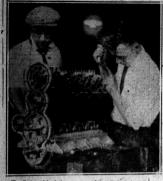
The first model of the new type four-cylinder, alr-copied, overhead valve-motor for airplanes developed and built by Chevroled Brothers Manufacturing Company in their Indianapolis plant for the Mogndoville Airplane Corporation is shown on the motor block a few mours before it was finally askembled, tested and shipped early Friday
