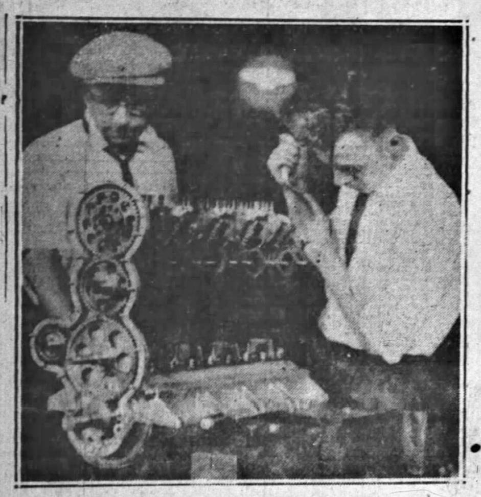
The first model of the new type four-cylinder, air-cooled, overhead valve motor for airplanes developed and built by Chevrolet Brothers Manufacturing Company in their Indianapolis plant for the Moundsville Airplane Corporation is shown on the motor block a few hours before it was finally assembled, tested and shipped early Friday to Moundsville, W. Va.
